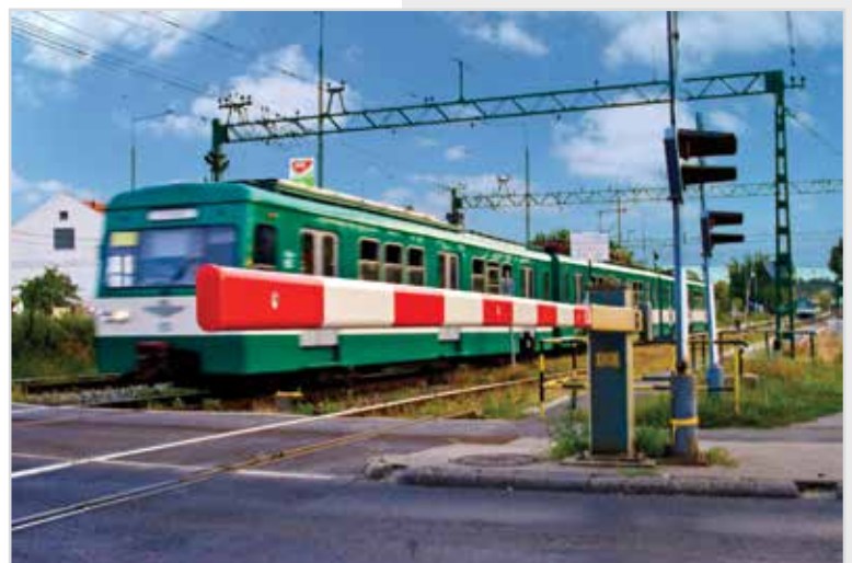
A HSH-03 type barrier drive at Cinkota station of BKV-HÉV suburban railways
