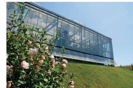
EXTERIOR OF AN ORGANICA WWTP
